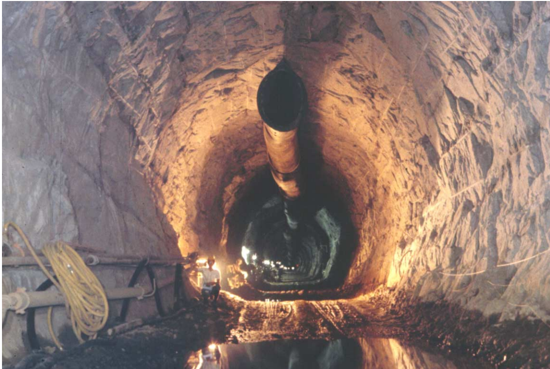
Figure 16.5: Results achieved using well designed and carefully controlled blasting in a 19 foot diameter tunnel in gneiss in the Victoria hydroelectric project in Sri Lanka. Photograph reproduced with permission from the British Overseas Development Administration and from Balfour Beatty - Nuttall.
