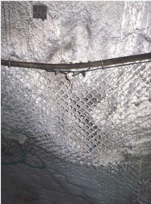
Figure 15.7: Chainlink mesh, while very strong and flexible, is not ideal for shotcrete application because it is difficult for the shotcrete to penetrate the mesh.
