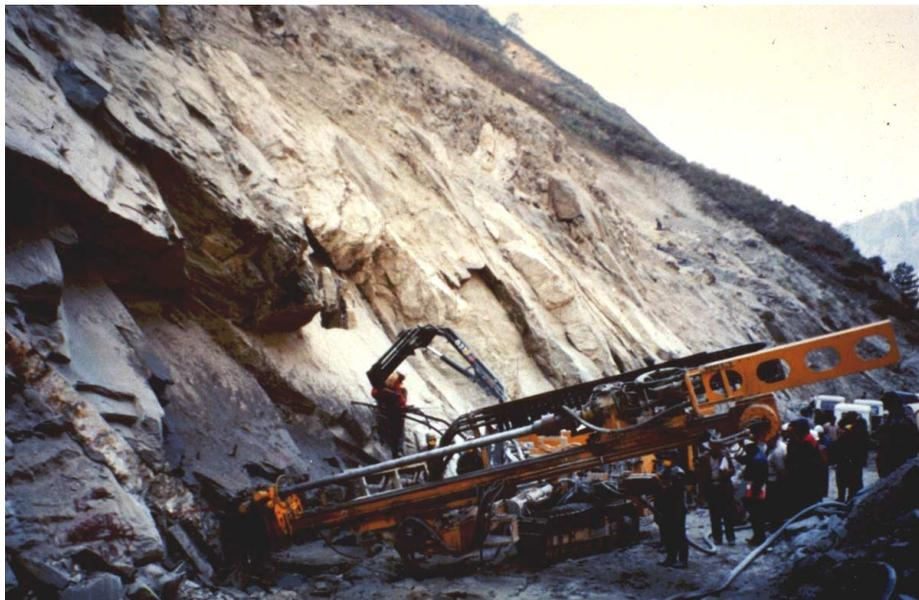
Figure 14.16: Drilling machine for the installation of 40 m long reinforcing cables in 150 mm diameter holes in a dam excavation.
