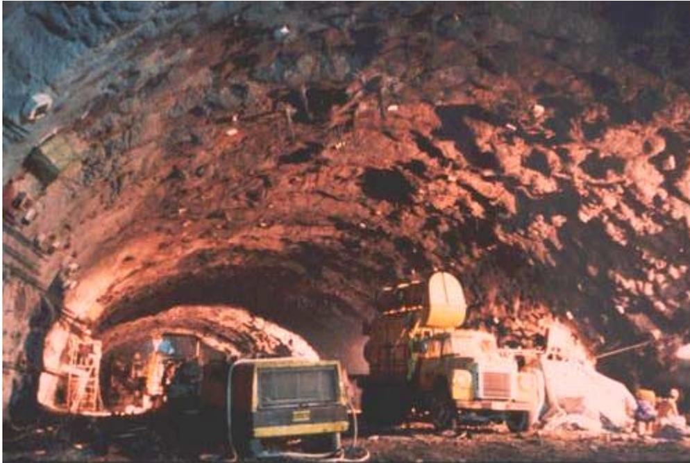
Figure 13.19: Cables and shotcrete were used to support the roof of the power cavern in the Mingtan Pumped Storage Project in Taiwan.
