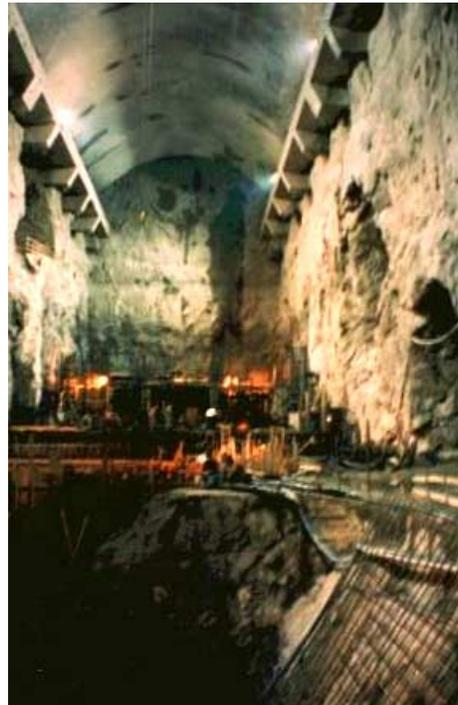
Figure 13.10: Example of anchored crane beams in the underground powerhouse cavern for the Thissavros Hydroelectric project in Greece. In this case the beams shown were used for a construction crane and concrete columns were added later to carry the full crane loads.
