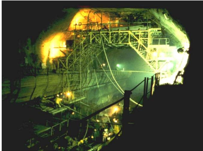
Figure 13.8: Example of a cast in place crane beam in the Drakensberg Pumped storage project in South Africa. The beam is supported against a vertical face of interbedded sandstone, siltstone and mudstone by means of stressed and grouted cables. A temporary construction crane that was used to access the roof is shown in the photograph.
