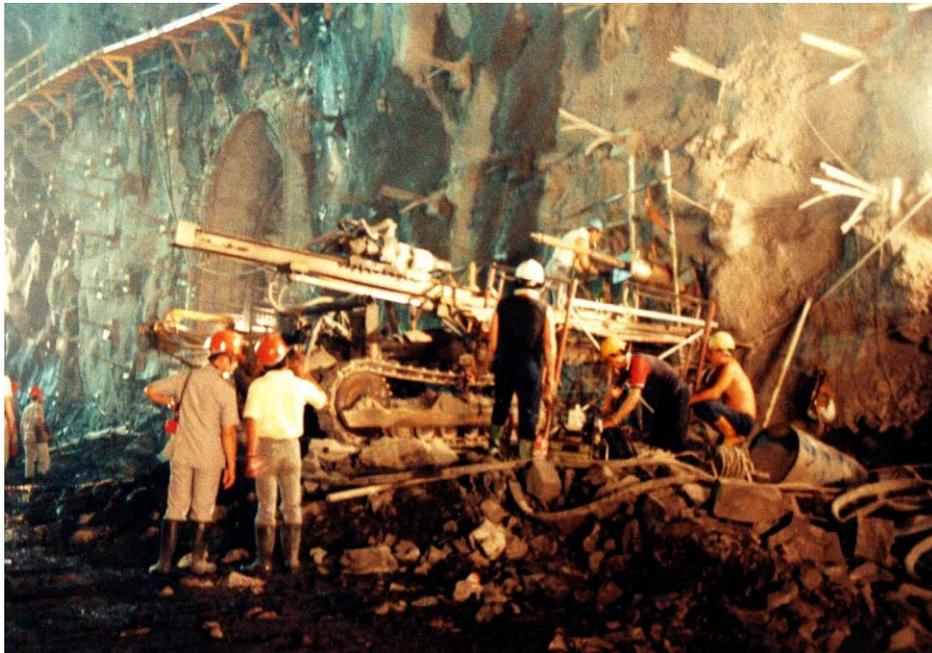
Figure 14.30: Installation of cables in the sidewall of the power cavern in the Mingtan Pumped Storage Project in Taiwan.
