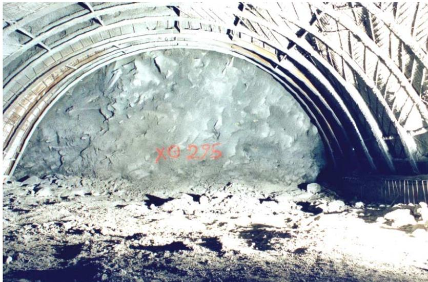
Figure 10.14: Top heading supported by cables and rockbolts and light steel sets.
