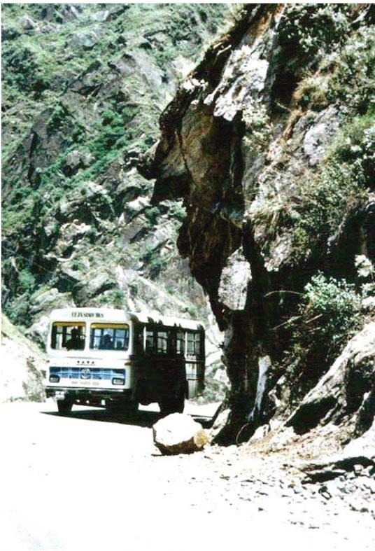
Figure 9.1: A rock slope on a mountain highway. Rockfalls are a major hazard on such highways.
