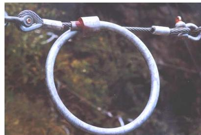
Figure 9.5: Details of a rockfall net system manufactured by Geobrug of Switzerland.
