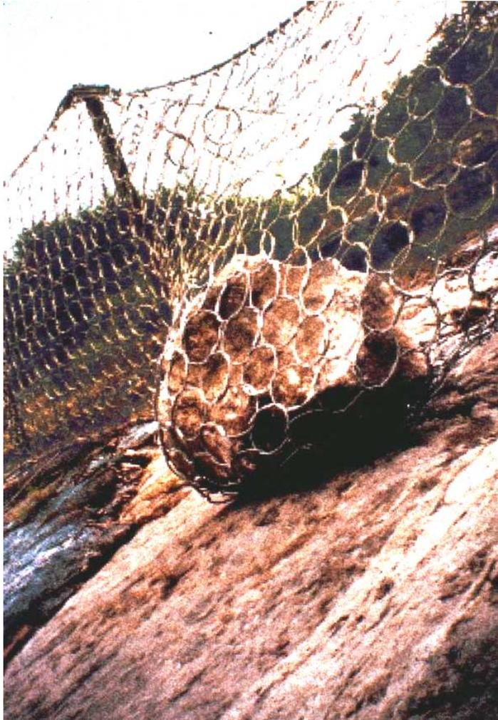
b: Geobrug ring net shown restraining a boulder. These nets can be designed with energy absorbing capacities of up to 2500 kNm which is equivalent to a 6 tonne boulder moving at 20 m per second.
