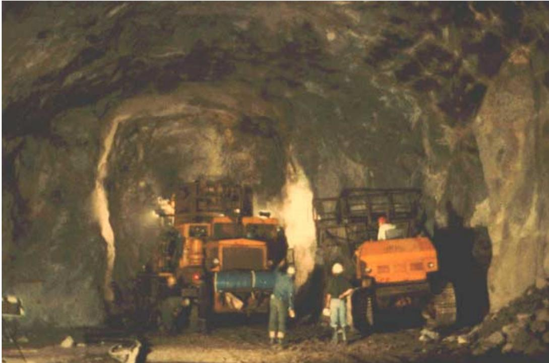
Figure 6.4: A 6 m wide heading driven ahead of the tunnel face to permit pre-reinforcement of potentially unstable wedges in the roof. The seven-boom jumbo is seen working in the heading.
